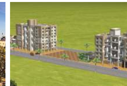
SHRI VENKATESH NISARG Commercial Spaces & 1,2,3 BHK Apartments, Vadgaon BK, Pune
